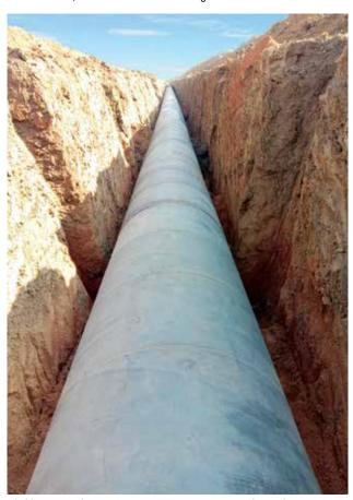
1500 mm dia MS Pipeline laying work for Bilaspur Water Supply Scheme, in Chhattisgarh.
