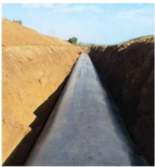
2028 mm dia MS pipeline laying work for Narmada Water Resources, Water Supply Scheme & Kalpsar Department, Palanpur in Gujarat.
