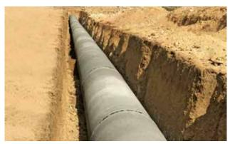
1700 mm dia PCCP pipeline laying for KPCL Bellary Thermal Power Plant, in Karnataka
