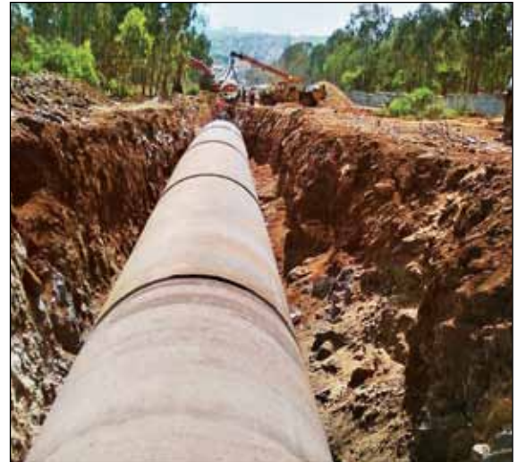
1825 mm dia duly lined & outcoated M. S. Pipe for W.S. Project Phase-II BWSSB-W5d Project Bangalore
