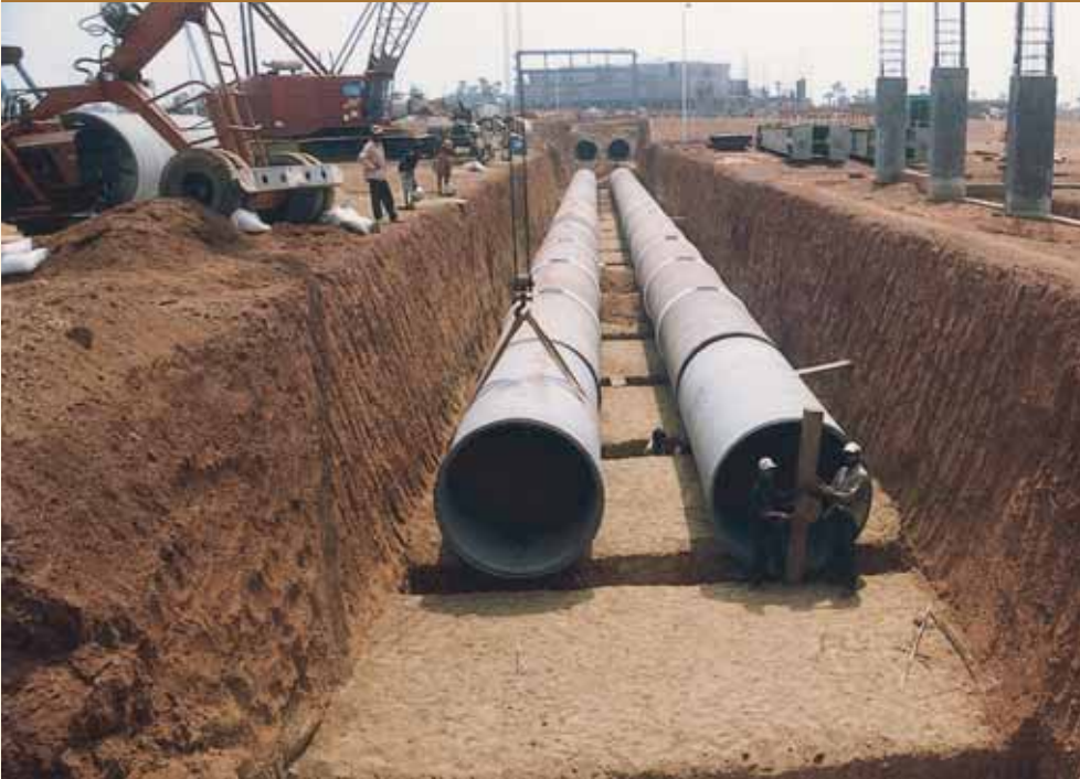
1800mm dia. BWSC cooling water circulation twin pipe line at samalkot, for 220 MW, BAPL, combined cycle power project of BSES at J.D.A. Peddapuram near Kakinada, Andra Pradesh.
